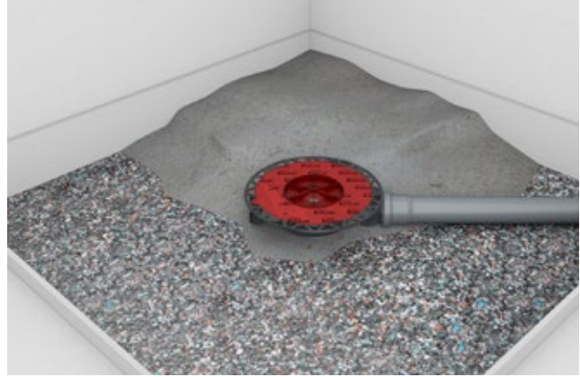
Step 2: The area is now filled with screed.
