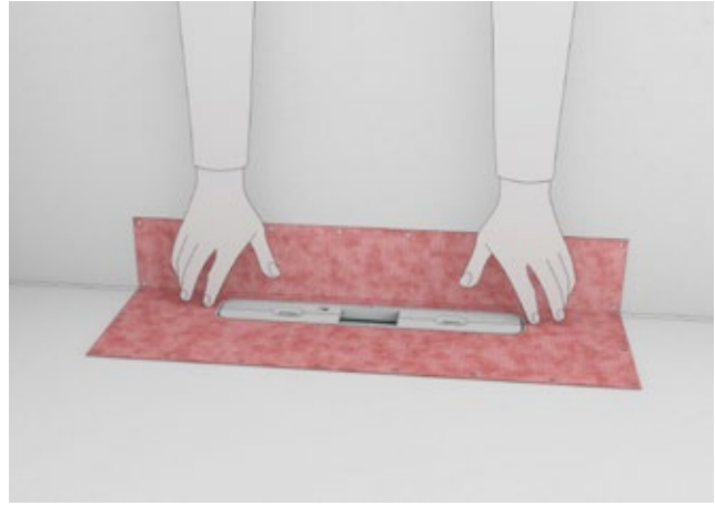
Step 4: Sealed with a click: once the screed has been installed, the first part of the bare-wall protection is removed from the drain and the sealing sleeve supplied is inserted via the click mechanism. The shower area can now be sealed and tiled.
