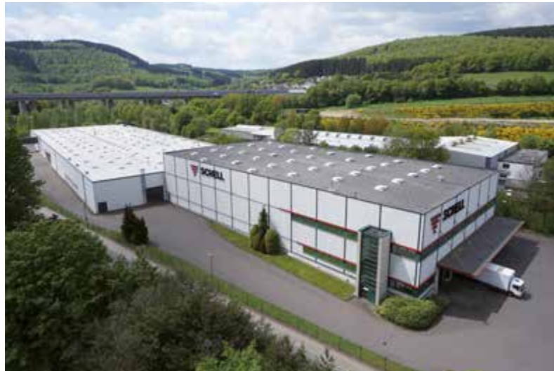
Plant 2 Production with logistics centre
